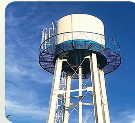
OVERHEAD WATER TANK
